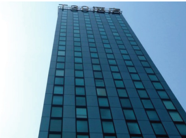
December 2011, the T30 Hotel constructed in 15 days. Photo: Lloyd Alter.
